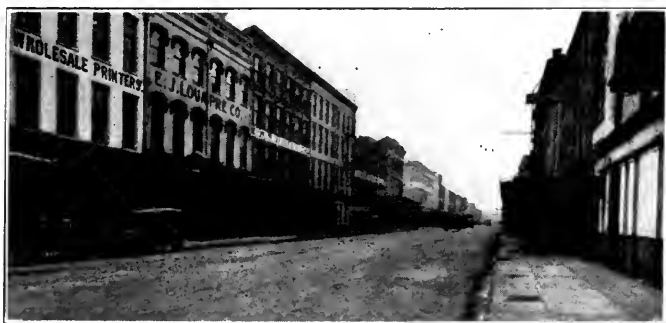
POYDRAS STREET COMPLETED
